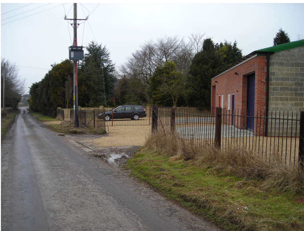
Figure 4: Photograph of the units and two access points to Bytham Road
